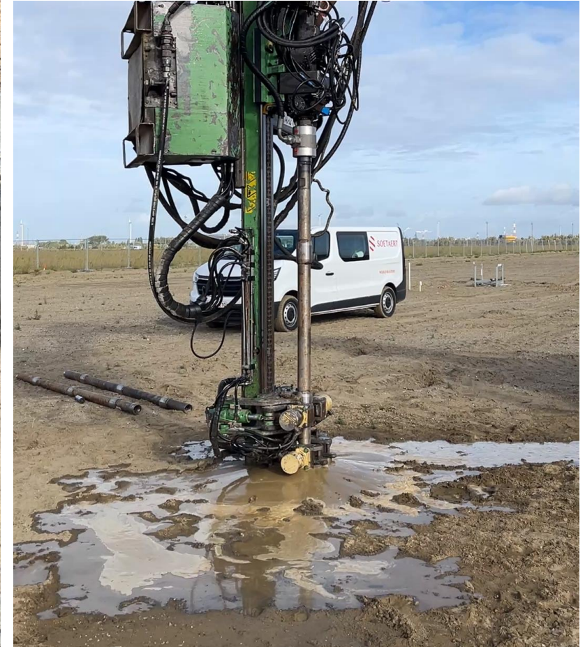
Unsuccessful injection due to the limiting geological parameters
